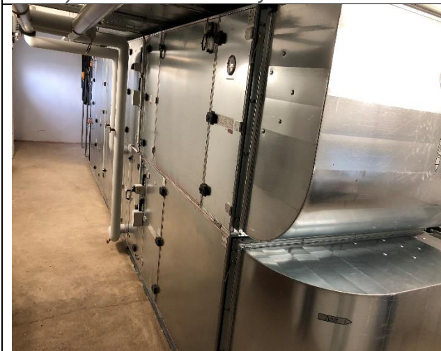
view of the new ventilation system
