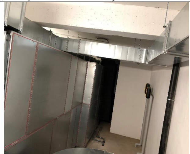
view of the new ventilation system
