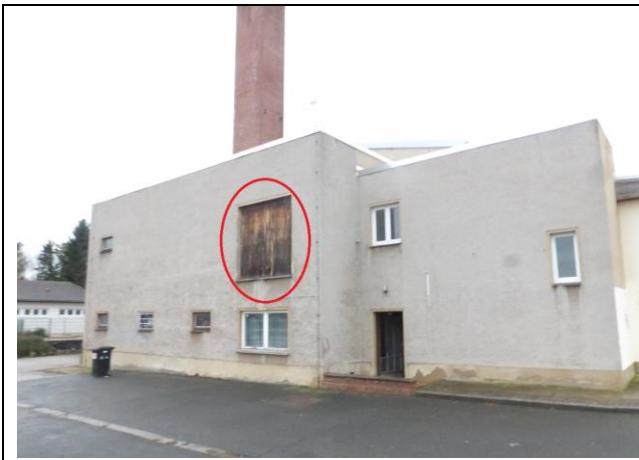
Central heating and ventilation unit. The large opening in the ventilation centre facilitates the dismantling of the old system and the installation of the new system.
