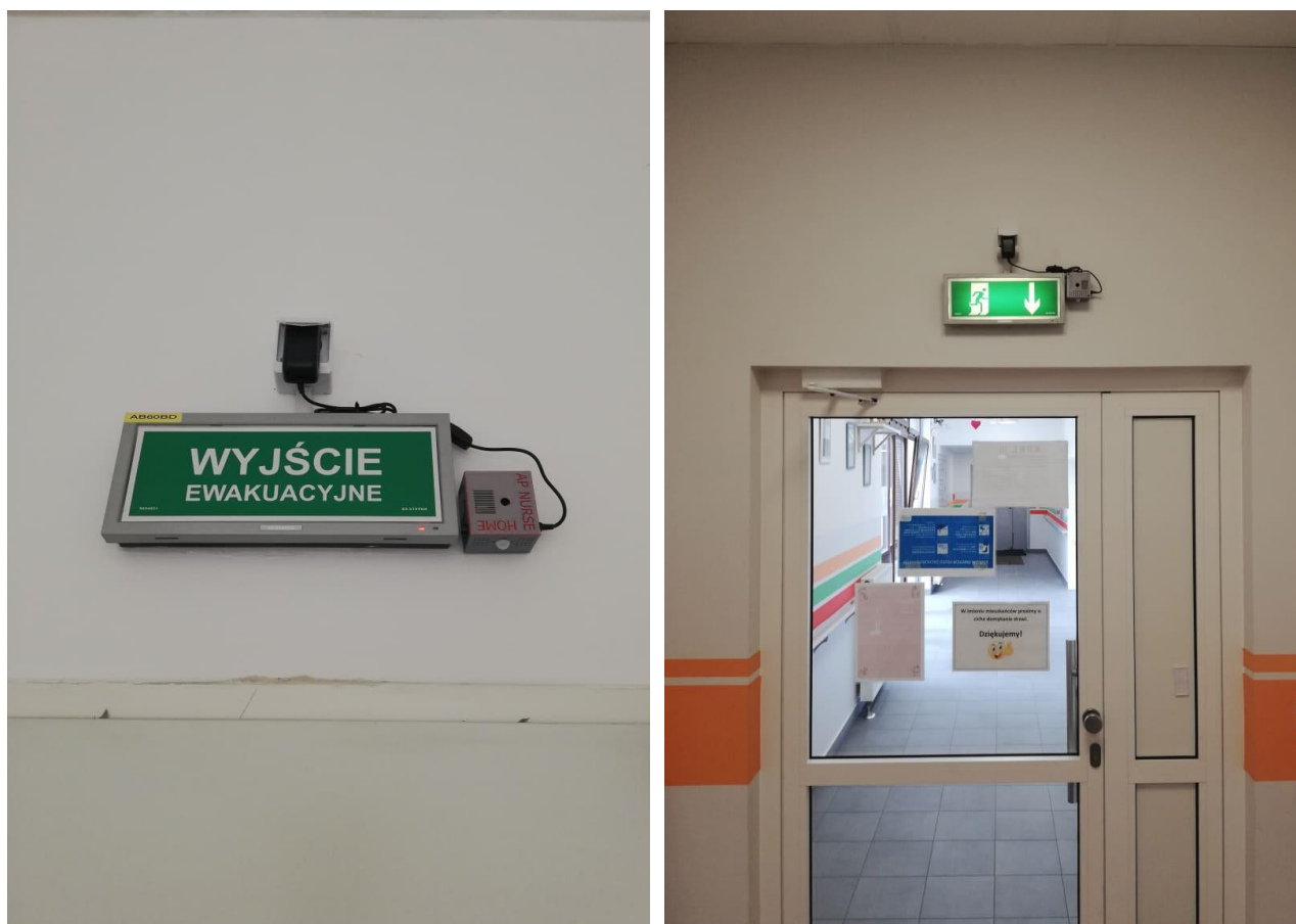
Figure 19. AP4-H-003 device installed above the door of the orange exit from the main corridor
