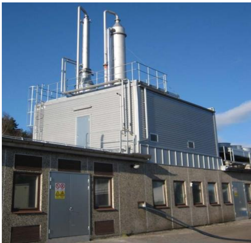
Biogas upgrading plant Gothenburg, Sweden with a raw biogas capacity of 1600m 3 /h (Source: Cirmac)
