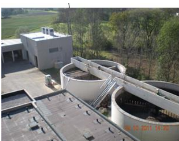
Fig. 5 sludge storage tank prior processing
