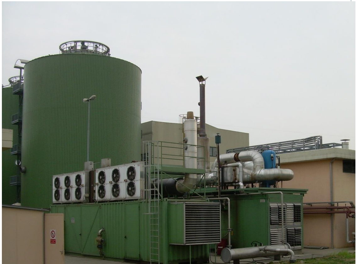
Anaerobic Digestors and CHP units
