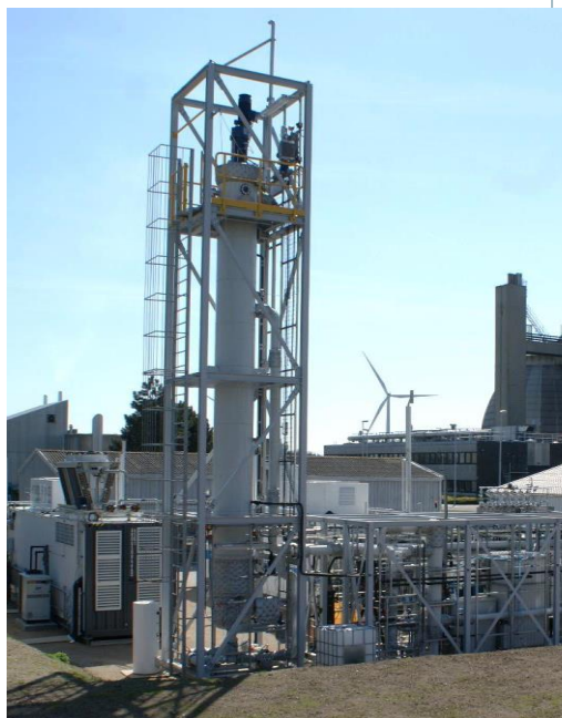
biomethanation reactor using CO 2 produced in the digesters to perform biogas-upgrading for gas grid injection
