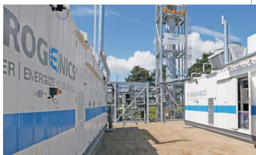
electrolyzer from hydrogenics delivering hydrogen to the BioCat methanation plant and oxygen to the waste water treatment plant
