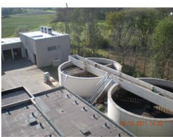
Fig. 5 sludge storage tank prior processing
