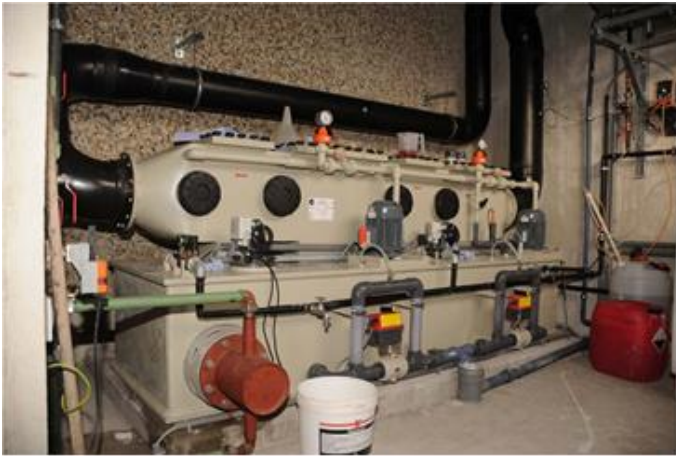
Fig. 9 Biofilter
