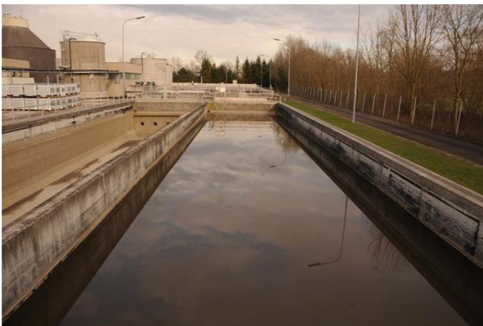
Fig. 1 primary sedimentation tank
