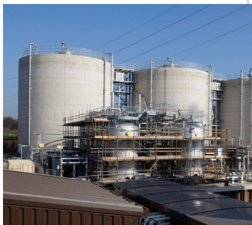
Advanced Digestion plant under construction including twin stream Cambi THP - PHOTO by Steve Mayes - Courtesy of Northumbrian Water Ltd ( www.waterprojectsonline.com/case_studies/2012/Northumbrian_Howdon_2012.pdf )
