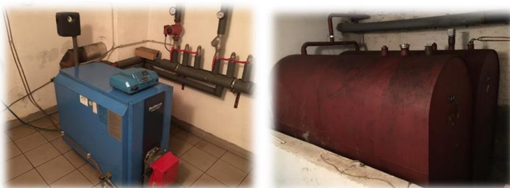
Figure 7: Existing inefficient old heating oil boiler
