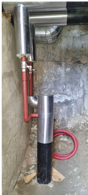
Figure 11: Construction work - connection of the new pipeline to the primary network
