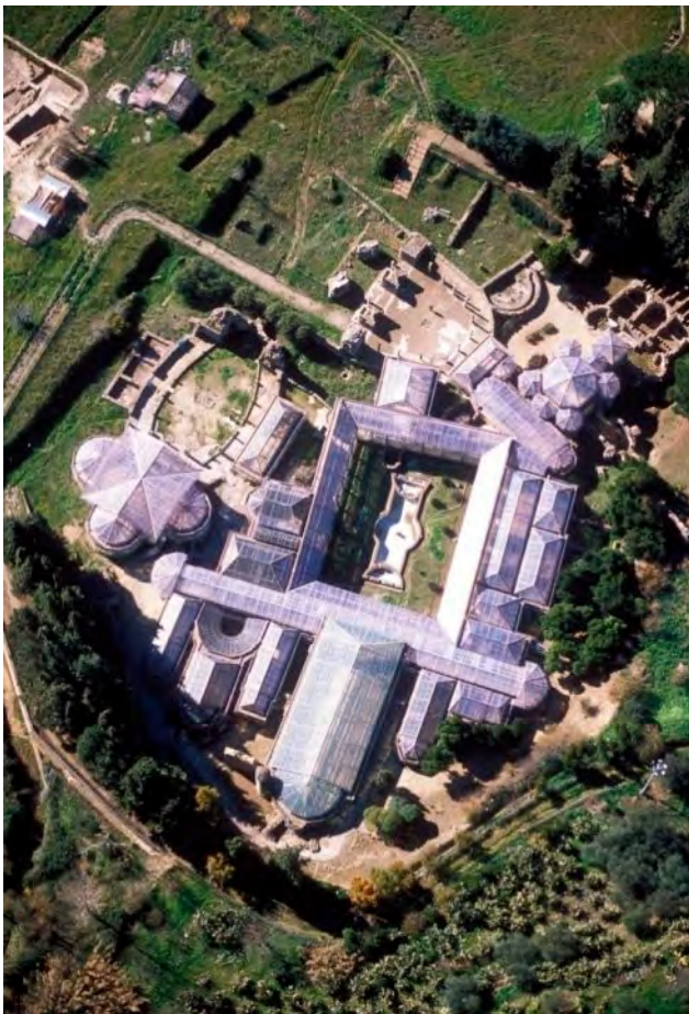
Villa Romana del Casale, aerial view, intervention by Arch. Minissi.
