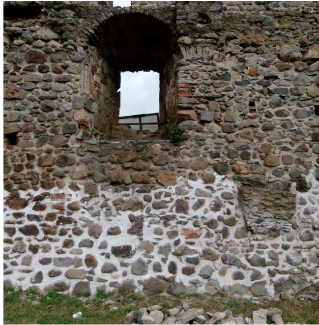
Poor craftsmanship in the initial stage of the northern ramparts conservation expressed in enormous areas of mortar signaling lack of wedging with stone.
