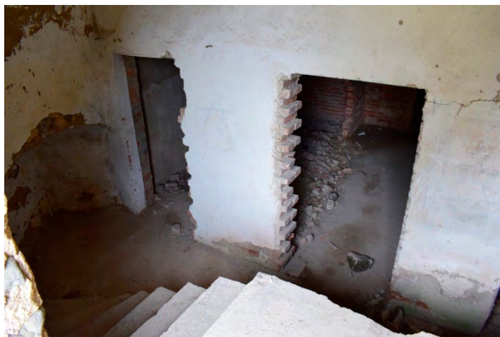
Ground floor of southeast tower with a new arrangement of the inner space
