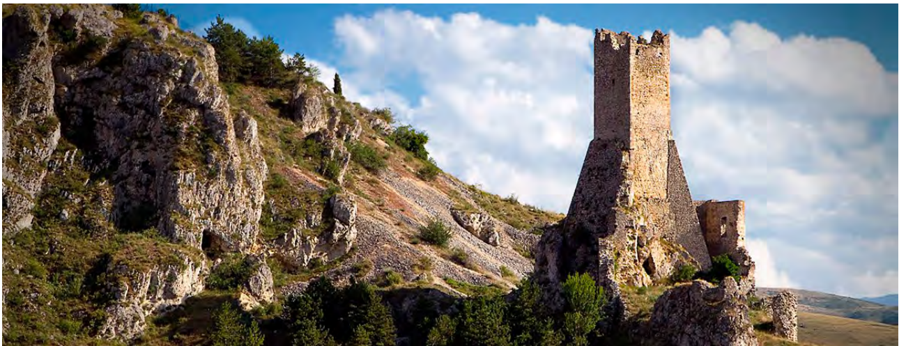
Tower of Pescina, the medieval structure built in a strategic position to control the mountain pass, has resisted the abandonment and the devastating earthquake of 1915.
