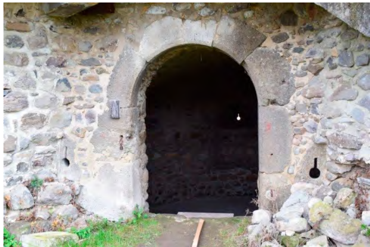
Entrance to the ground floor of the southwest tower. In the photograph from the restoration time, it is visible that the whole wall in which the doorway and loopholes are set was not preserved and has been created anew.
