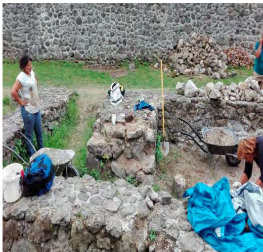
A decomposed segment of masonry restored with technology from the 1960s re-restored in lime technology.
