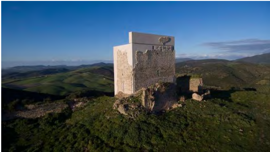
An intervention that has been much discussed, the restoration of the Castle of Matrera in Spain
