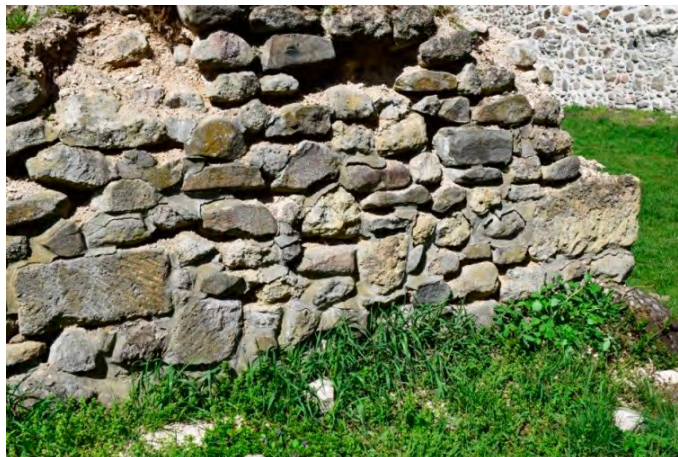
A fragment of a wall showing the decomposed original substance behind the cement mortar
