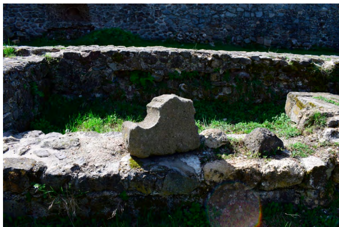
A cement based cap on the decomposed original substance of the excavated church foundations
