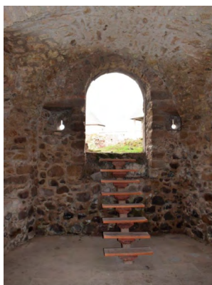
The doorway shows the original level of the ground in the southwest tower. All the masonry below this level is unearthed foundations.
