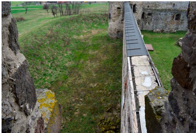
Temporary covers on the top of northern rampart, partially destroyed by the winds.
