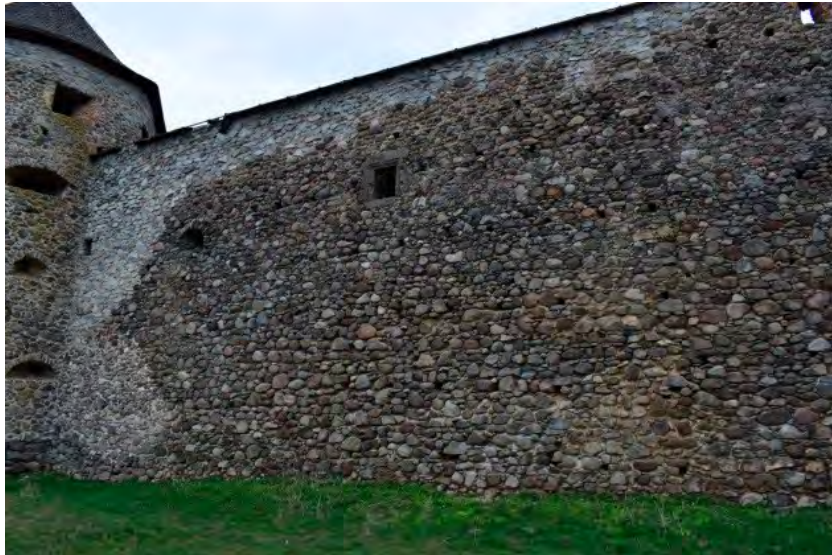
A section of southern rampart showing the recognizable addition of the masonry.
