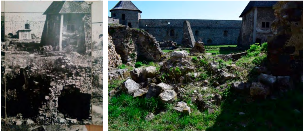
The same original historic construction in the photographs made during the restoration and today. The decline of mass due to no protection is clearly visible.
