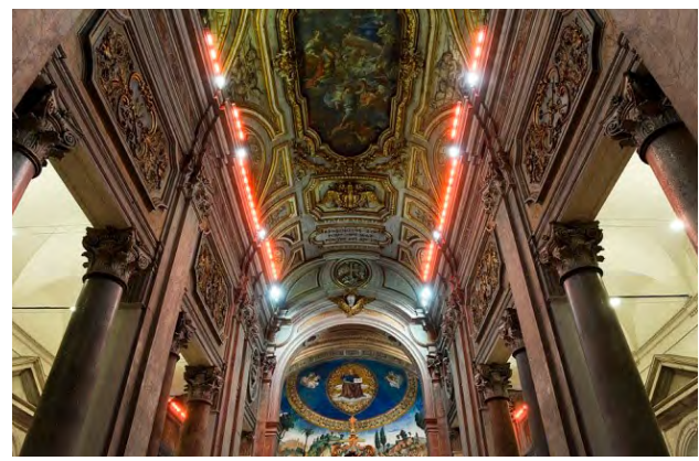
Electric radiation heating with intermittent operation. Basilica S. Croce in Gerusalemme, Roma.
