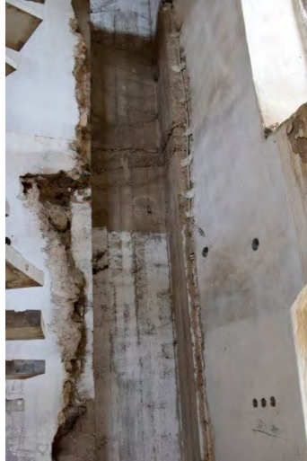
Shaft for plumbing inside northeast tower
