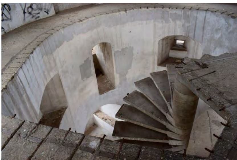
New utility constructions done in concrete to be distinguished from original substance of the heritage.
