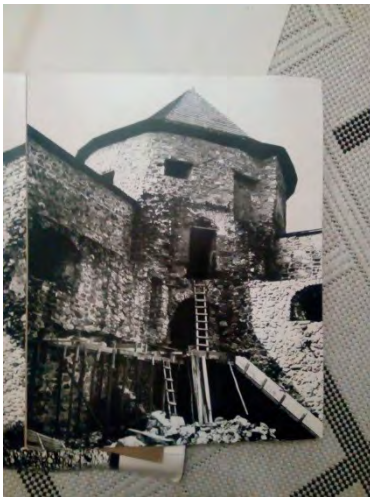
Entrance to the ground floor of the southwest tower. In the photograph from the restoration time, it is visible that the whole wall in which the doorway and loopholes are set was not preserved and has been created anew.
