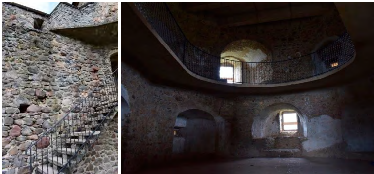
Contemporary safety railings applied on the concrete platforms and stairways made in the 1960s.
