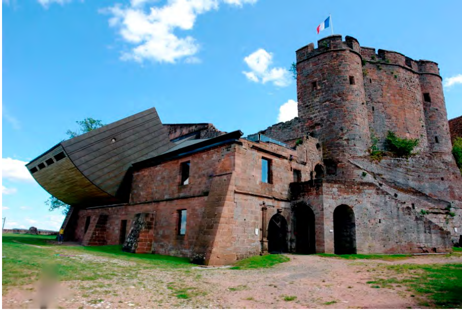
Intervention on Lichtenberg Castle by Andrea Bruno. In this case, a new organic unit is sought, in which the relationship between the old and the new one comes into question
