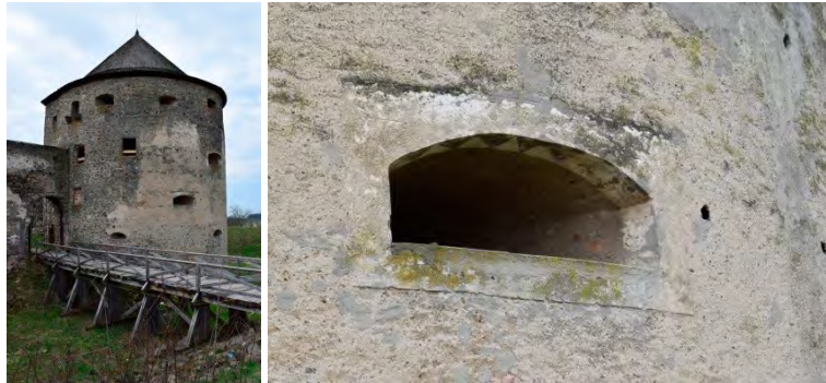
Roofed northwest Tower and a detail of the preserved decorations on plaster around one of the loopholes
