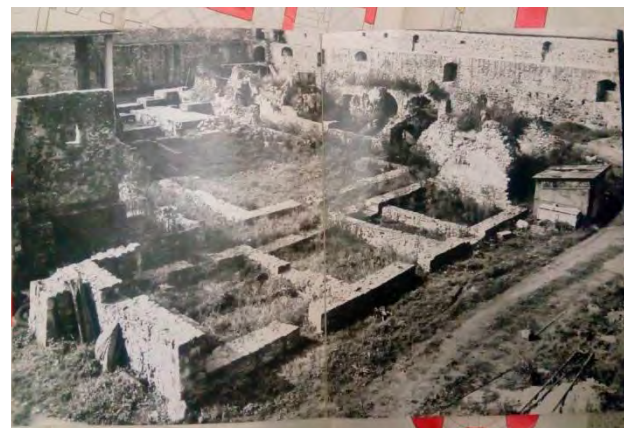
The comparison of the preserved mass in the time of restoration and today. The decline of the original mass is in great part due to the unfinished process of restoration. The contrast between the roofed objects and the ruins of monastery are the result of mixed restoration approach.
