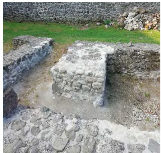
A decomposed segment of masonry restored with technology from the 1960s re-restored in lime technology.
