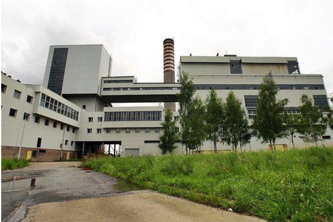
Photo 2. Abandoned building of the former power plant
