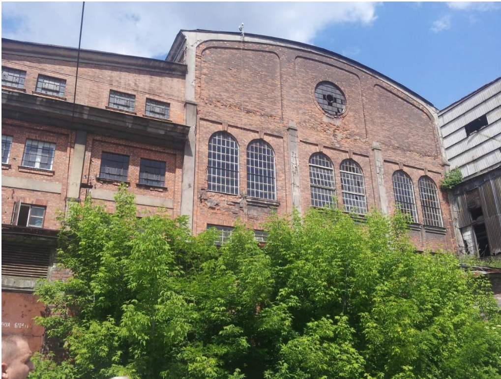
Photo 5. Deteriorated power plant
