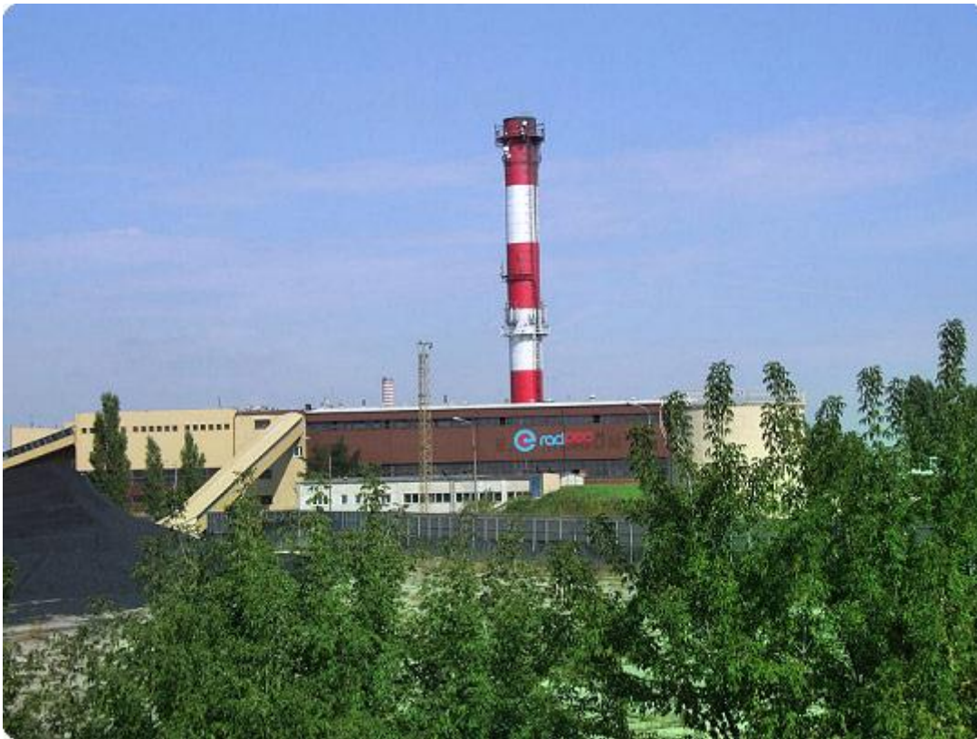
Photo 3. Power plant „North”
