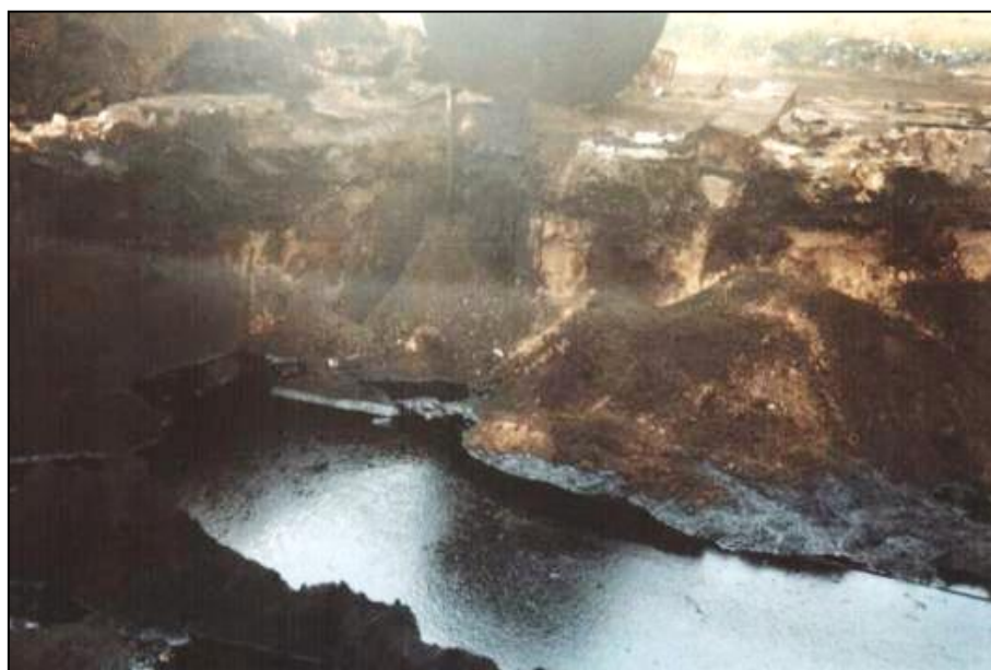
Fig. 26. Unveiling tanks with pouring creosote into the ground (2005) (by W. Irmiński)
