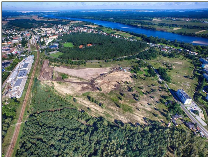
Fig. 11. Brownfields in Solec Kujawski, bird's-eye view (property of the commune)
