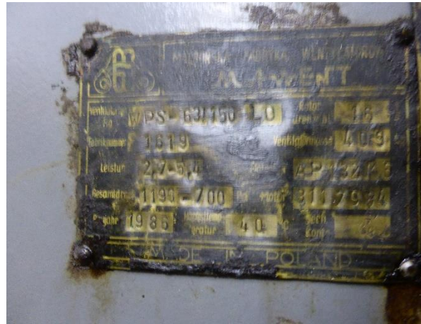
Ventilation system nameplate
