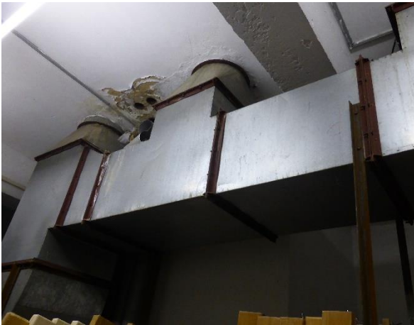
View of the existing ventilations system
