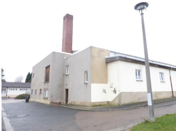
Central heating and ventilation unit
