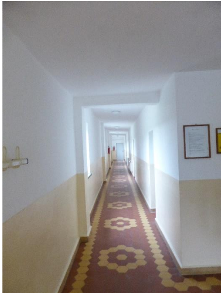
Interior view of the floor
