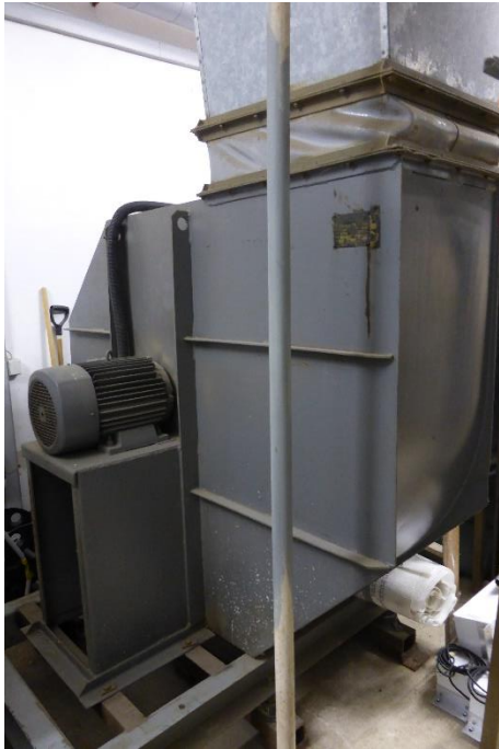
View of the existing ventilations system
