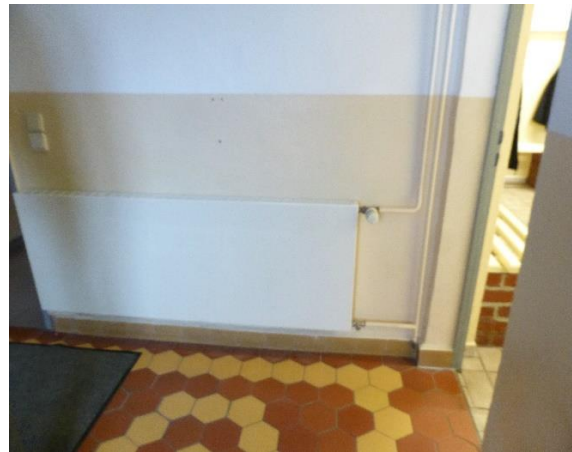
Radiator in the floor
