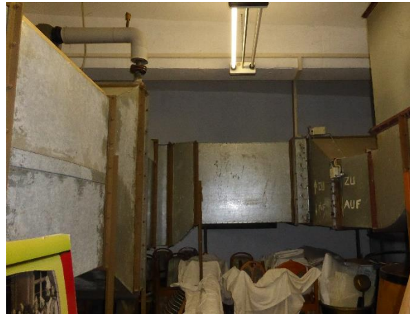
View of the existing ventilations system
