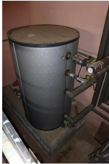
hot water tank
