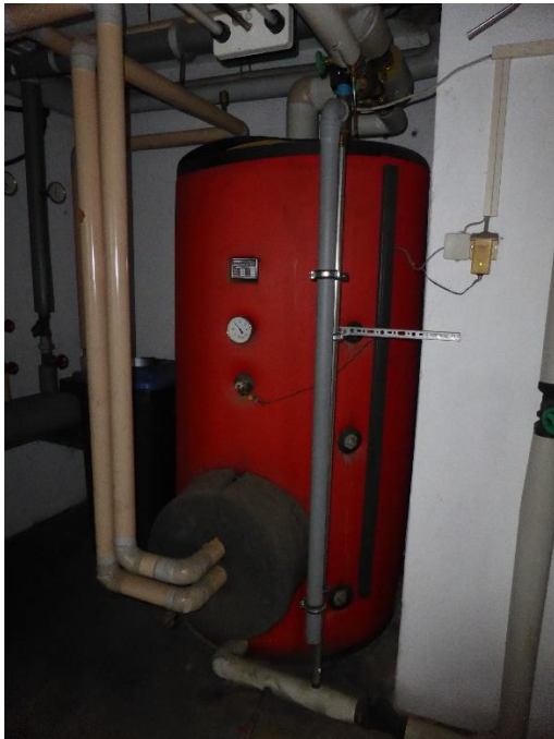
hot water tank
