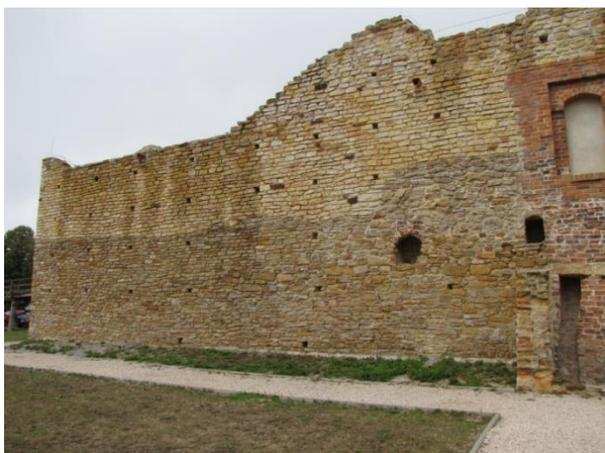
Fig. 17 . Reconstruction of substantial fragments of the wall with the material compatible with the historical one. (The castle of Inowłodz)
