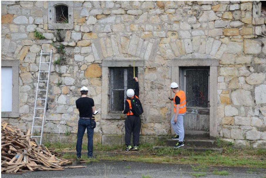
Photo 1 Measurements of the Donjon facade on the Kłodzko Fortress using the traditional method.
