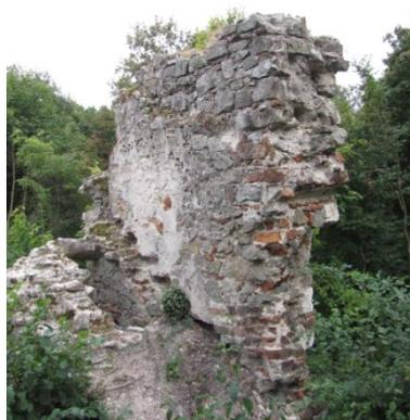
Photo9. Degradation of the wall due to the environmental factors /Międzygórz castle/
