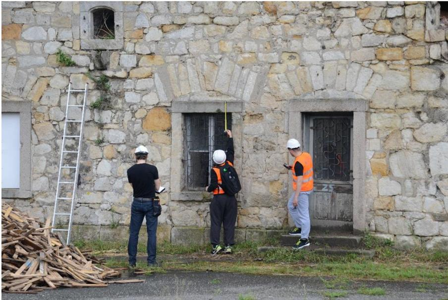
Photo 1 Measurements of the Donjon facade on the Klodzko Fortress using the traditional method.
