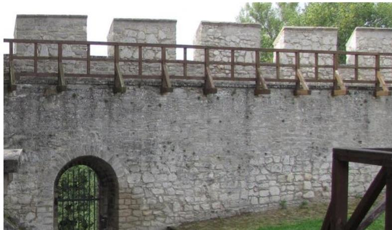
Fig. 19. Reconstruction of substantial fragments of the wall with the material compatible with the historical one)
