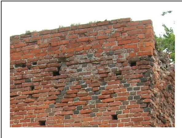
Fig. 22. Addition of the crown made of contemporary brick, on a type of mortar stronger than the original one. (The castle in Bobrowniki)
