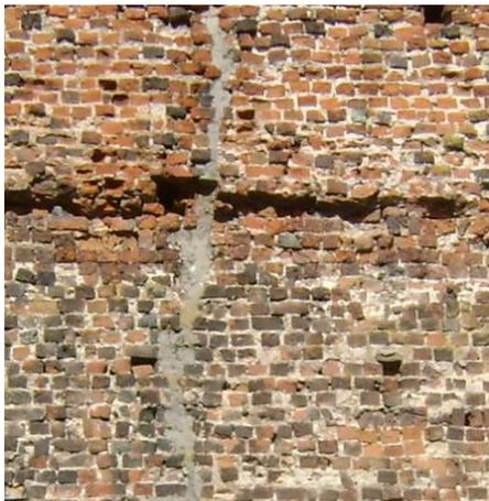
Photo 18. Injection into a crack with a cement mortar (photographer - Sylwester Zieńczuk) /castle in Liwa/
