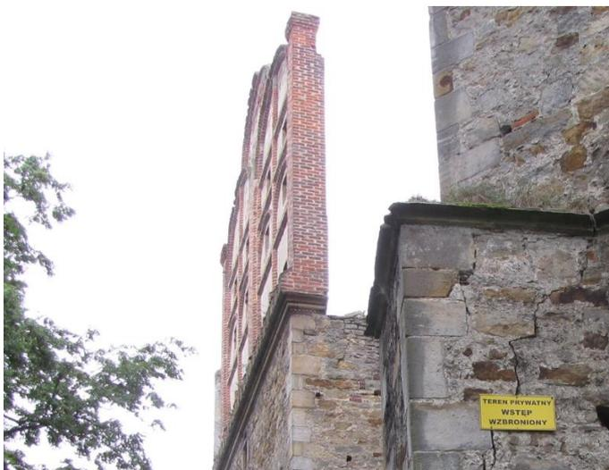
Photo14.Examples of cracks in a slender attic wall /castle in Drzewica/
