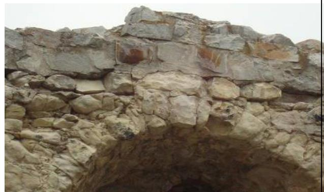
Fig. 21. Addition made of foreign material without the isolation layer. (The castle in Janowiec on the Vistula River)
