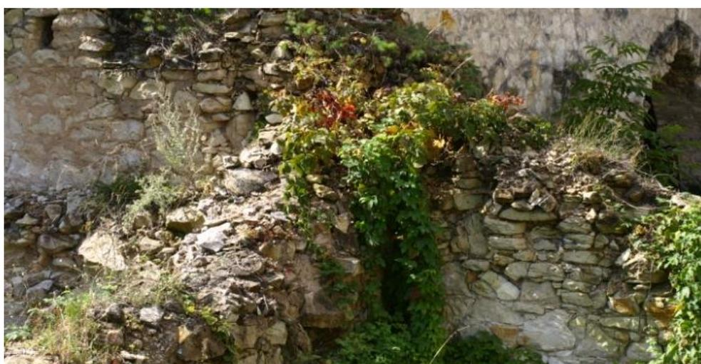
Fig. 16. A significant amount of annuals and perennials causing the degradation of the crown and the loss of legibility of the wall outline (contour).
