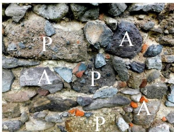
Fig. 2 Building material of the cloister (Cistercian Abbey): A - andesite, P - pyroclastic material
