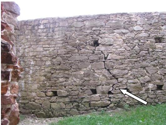
Photo12. Damage caused by uneven settlement /Krzyżtopór castle in Ujazd/
