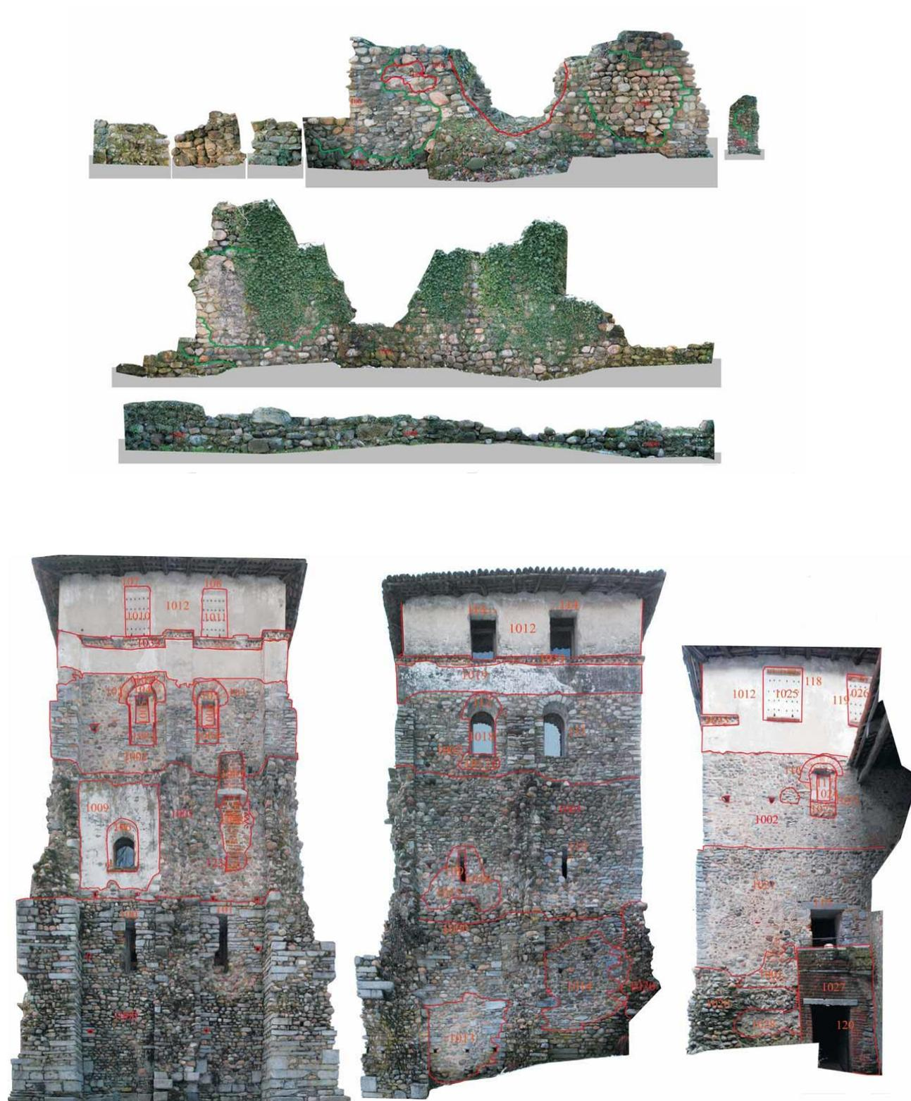
Picture 6: The analysis of the elevations and surveys aimed at the realization of the photo rectification of the structures (Archaeological Park of Castelseprio and Torba)
