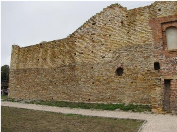
Fig. 17 . Reconstruction of substantial fragments of the wall with the material compatible with the historical one. (The castle of Inowłódz)
