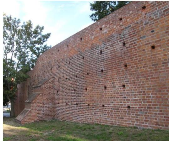
Fig. 18. Reconstruction of substantial fragments of the Wall with the material compatible with the historical one. (The castle of Łęczyca)
