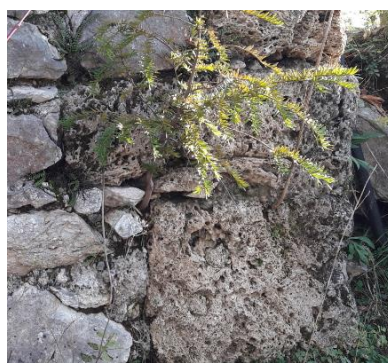
The sewn corner stones of the palace basement are made of tufa 306
