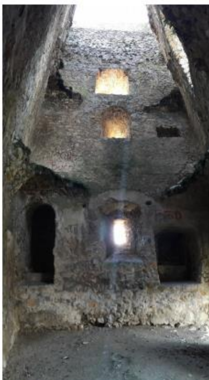
Image 84: Interior facade - S: 3 openings: two embrasures and a window
