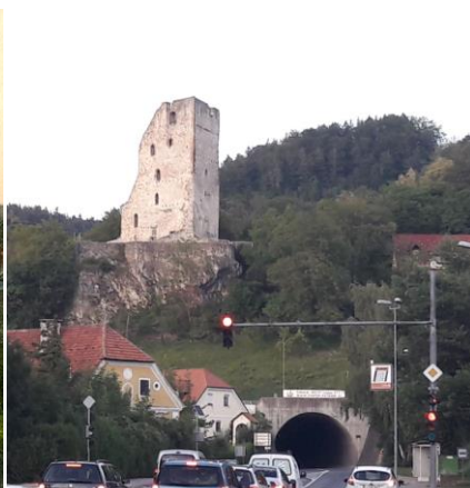
Šalek after renovation in 1990/91: parts of the ramparts, walls and tower were rebuilt, so the building regained some volume.
