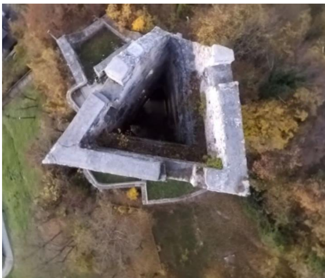
Aerial view of the top of the tower with a reinforced concrete crown: there may already be some cracks in the left corner – it is mandatory to constantly monitor the ruins. 360
