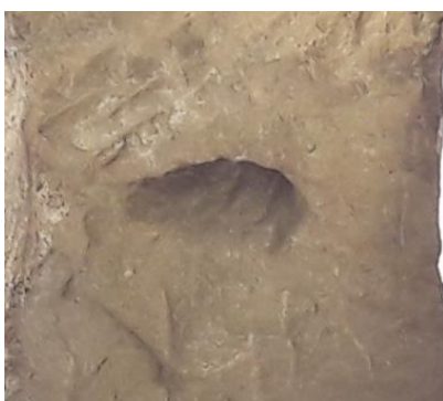
A sandstone lintel above the window on the ground floor of the tower, with a hole for a metal rod
