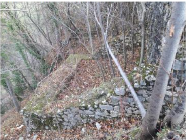
Image 90: Foundations of the building leaning on the northern side of the defensive wall
