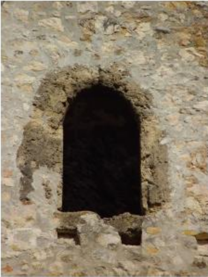
Image 92: Circularly finished door portal made of tufa.
