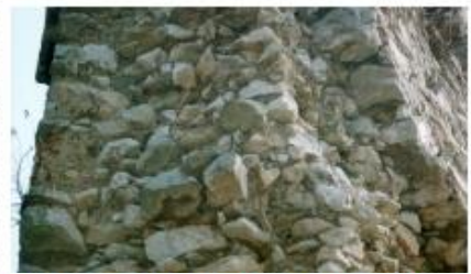
Image 100: building work of the opus emplecton type, clearly visible before the reconstruction: thick wall is made of three layers. First, two parallel walls were erected and the space between them was filled with stones and crushed rocks, quicklime was added and cooled with water - thus the filling changed into a monolithic conglomerate core which is however only poorly linked with stones in circumferential walls, which fall off.
