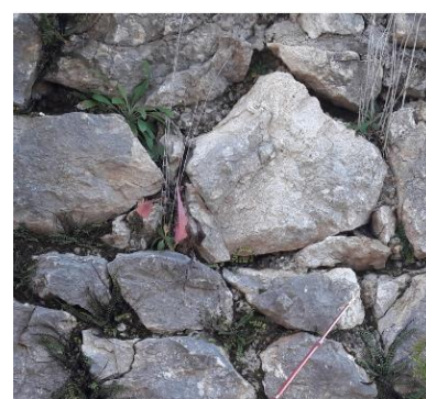
General limestone masonry
