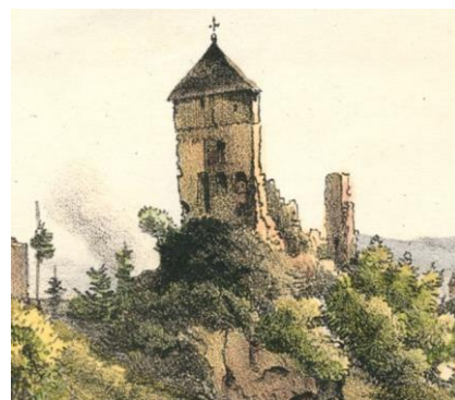
The view from the north. The triangular tower still has a roof.
