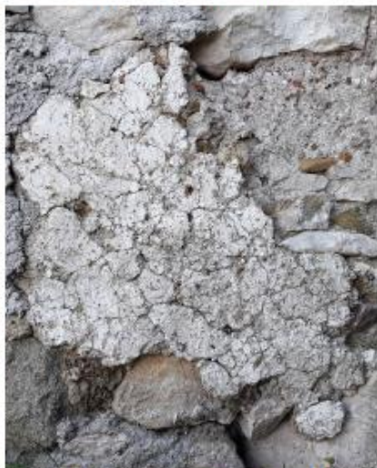
Image 99: White lime plaster on the tower facade facing the court yard
