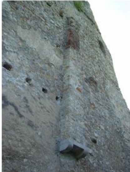
Image 93: Chimney on the eastern facade of the tower.
