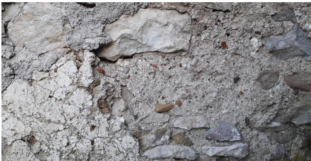
Crushed bricks in the castle walls mortar.
