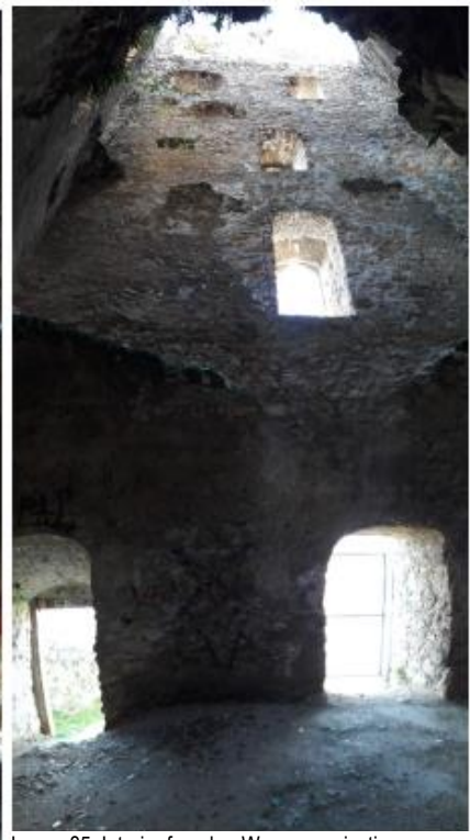
Image 85: Interior facade - W: communications were directed to the interior court yard. Two top windows are equipped with sedilias.
