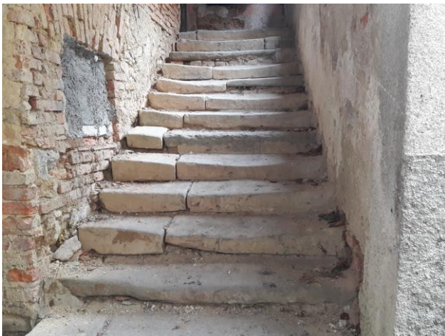
Stone stairs from Šalek, secondarily used at Turn Castle
