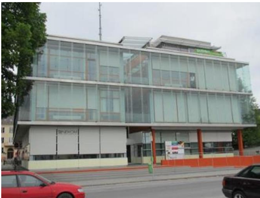
Figure 4.5: Situation test building
