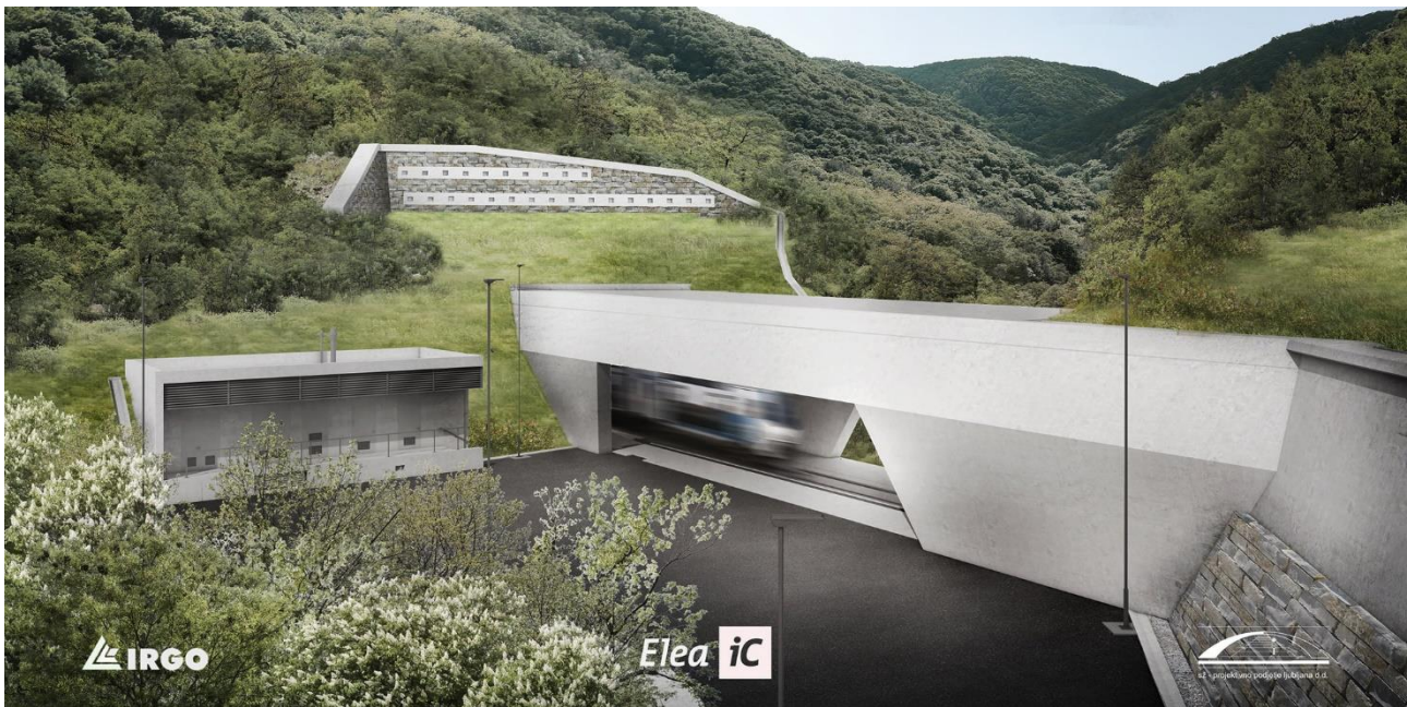
Figure 12 - Railtrack Divača Koper: New rail tunnel project (source: EleaIC)
