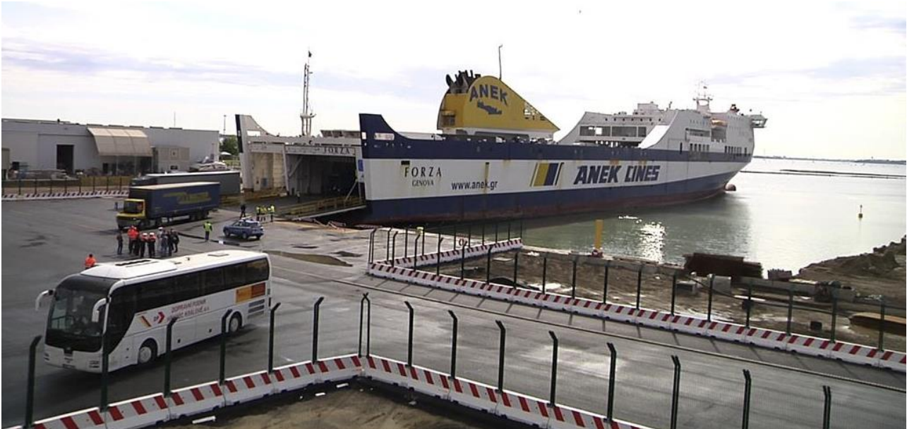
Figure 9 -Venice MOS Terminal Fusina
