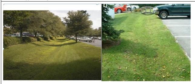
Figure 29. Grassy ditches and swales (source: RBMP, Urban rainwater management guide, 2015)
