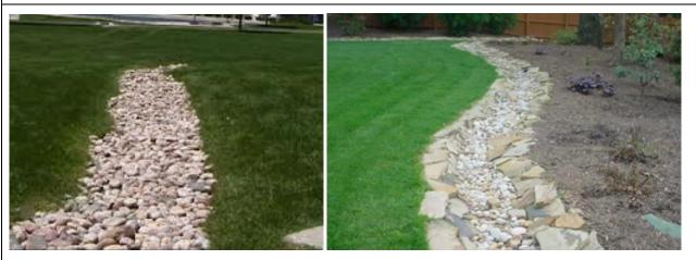
Figure 27. Infiltrating trenches (source: RBMP, Urban rainwater management guide, 2015)
