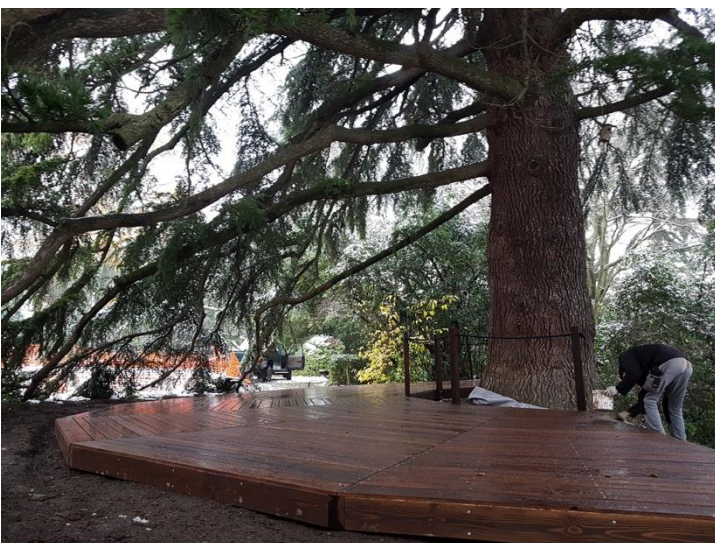
Details of the installation of the wooden platform around the big cedar
