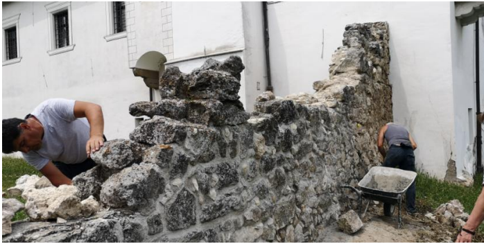
May 2019, wall works in progress
