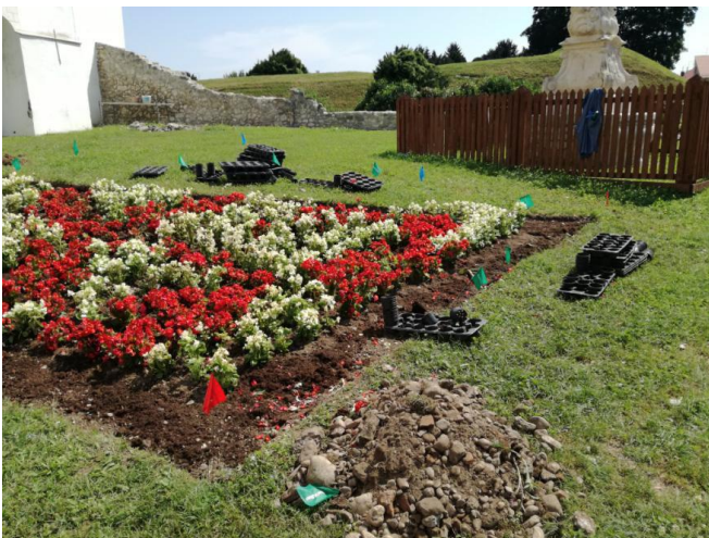
July 2019: Garden - works in progress
