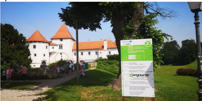
May 2019: Temporary panel announcement of works
