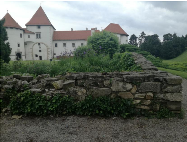
April 2019: Walls before works
