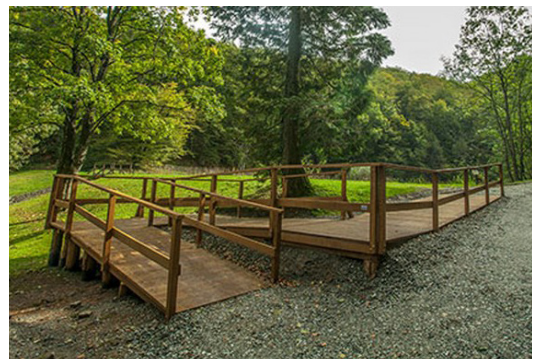
Wooden platforms for easier access for people with limited mobility.
