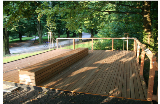
A wooden terrace and a handrail offer safe access to blind and visually impaired.
