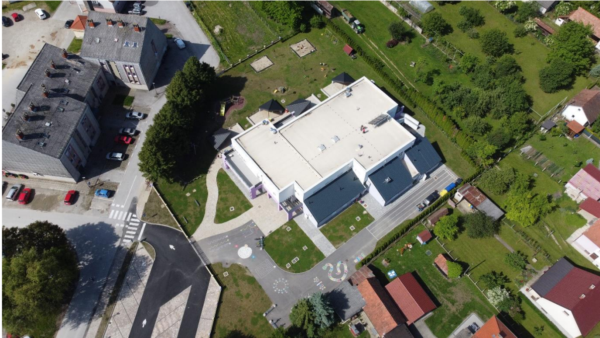
Image 2 Roof area of the Kindergarten "Fijolica" in Prelog
