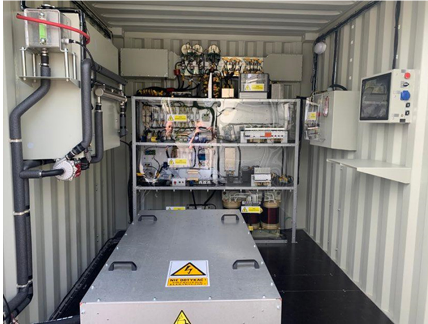
Figure 4: Battery-based electric energy storage; usage of a second-life traction battery from a trolleybus (Source: PKT Gdynia)
