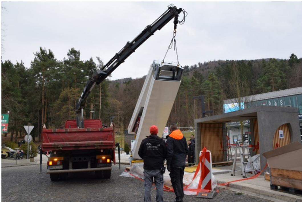
Figure 20: Installation of pantograph with a fast charger at cable car station in Maribor
