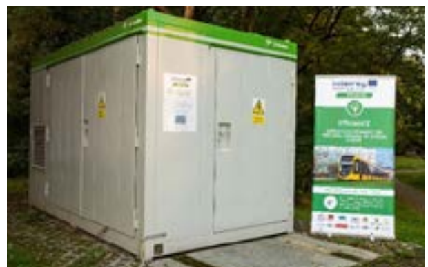
Abbildung 5: Batterie-Pufferspeicherstation in Pilsen (PMDP)
