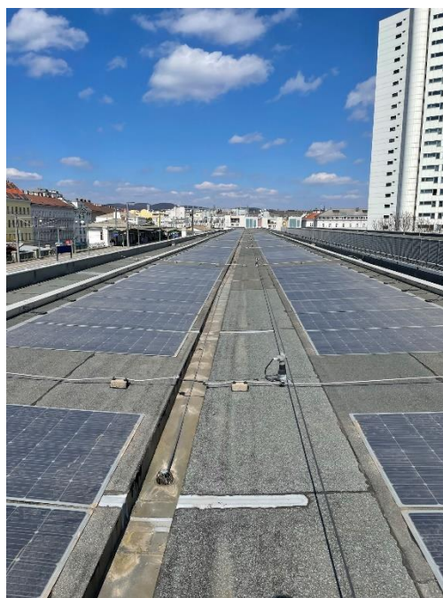
1. Figure: Light photovoltaic foils on the roof of a metro station in Vienna (source: Wiener Linien)
