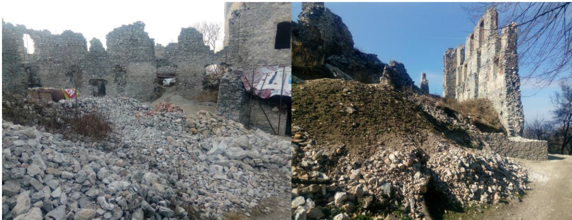
Figure 62 The abundance of manpower due to the program is sometimes difficult to manage in keeping everyone occupied. The solution of the coordinators is often to occupy the workers with digging the rubble which produces lots of historic building material. To sto
