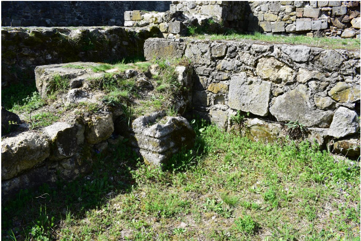
Figure 16 The foot of the pilaster carrying the cross vault of the church
