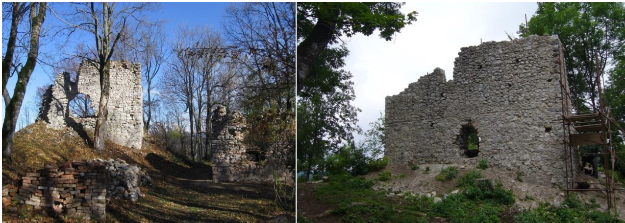
Figure 59 Restoration of the main tower of Castle Muráň which was done without any interference with the buried parts of walls. No details were recreated. The openings in the walls with unknown original shape were left in the form of cavern, only the masonry arou
