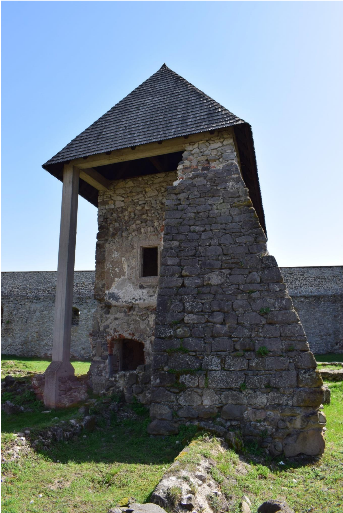
Figure 14 Chapel rebuilt from the original gothic presbytery of the monastery church
