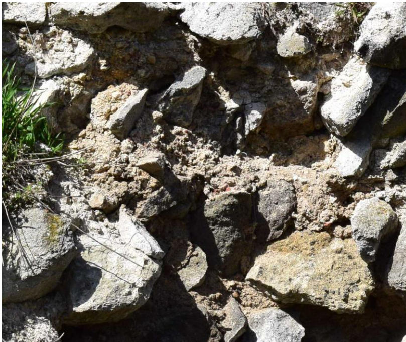
Figure 29 Detail of medieval mortar
