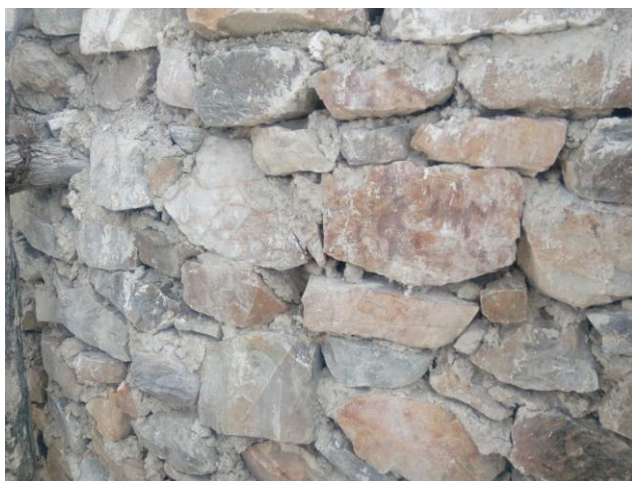
Figure 63 As the workers employed by the project are rarely professionals, they have no experience in the work they are hired for. This can undermine the professional work, and result in poorly executed craftsmanship. An example is this piece of masonry with no e
