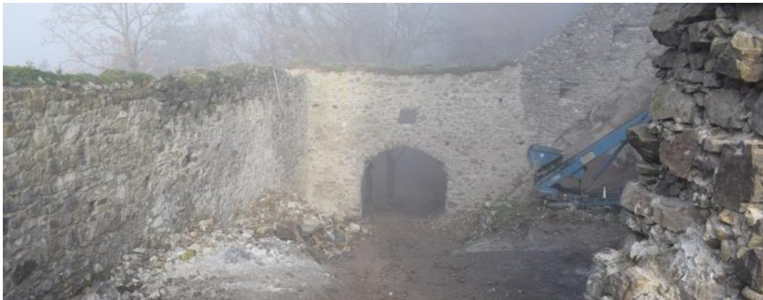
Figure 60 After a large portion of the ramparts of the inner part of the castle collapsed and filled the outer courtyard with rubble, it made the entrance gate impassable. Since there was no other access, the cleanup of the rubble had to be performed by hand, whi
