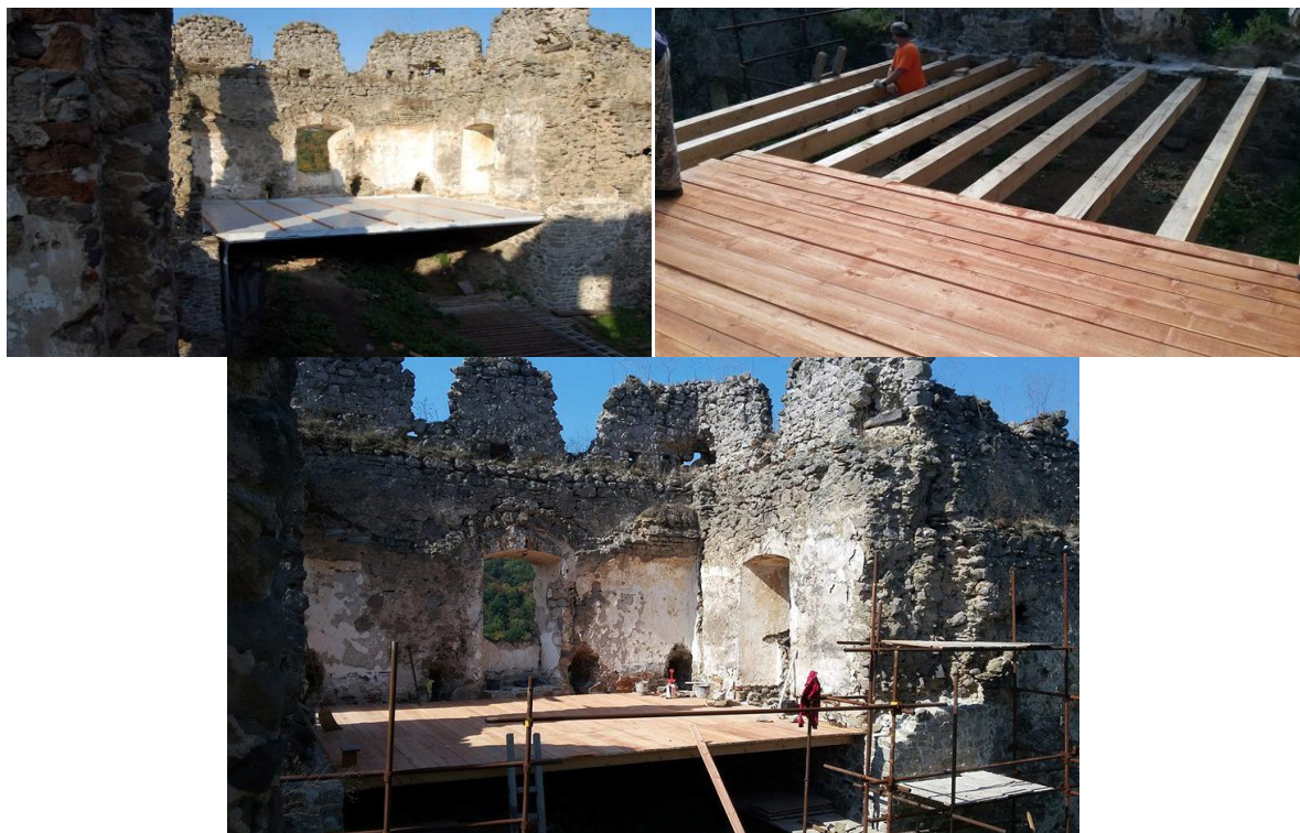
Figure 57 Roof on the defense tower of Castle Čabraď imitating a perished beam ceiling protecting original construction of the vault of the ground floor and redirecting the precipitation waters from the foot of the walls (it was causing a slow sliding of the tower)
