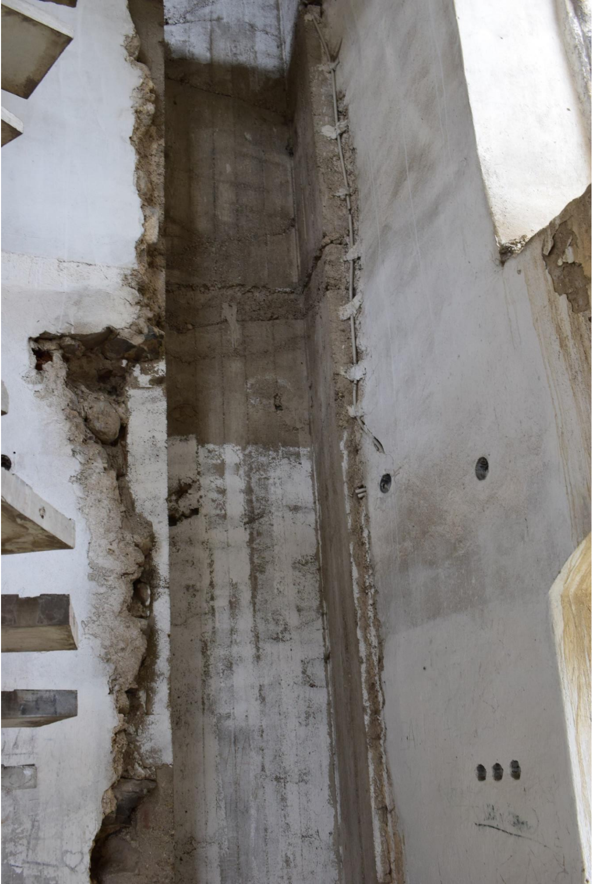
Figure 37 Appropriately done reconstruction of the fortifications with completions distinguishable from the original
