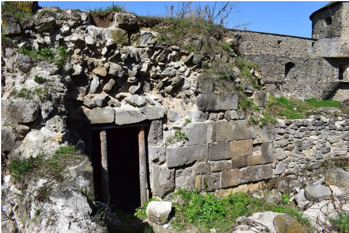
Figure 26 Block masonry with a core in a spiked weave in the northern towers of the monastery church
