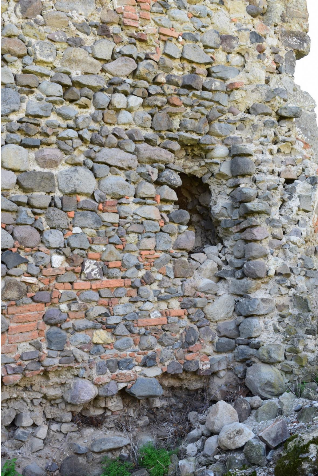
Figure 28 Detail of mixed masonry
