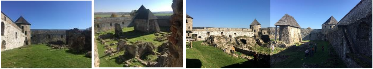
Figure 48 Pictures of the courtyard of the Bzovík castle (visual inspection in May 2018)
