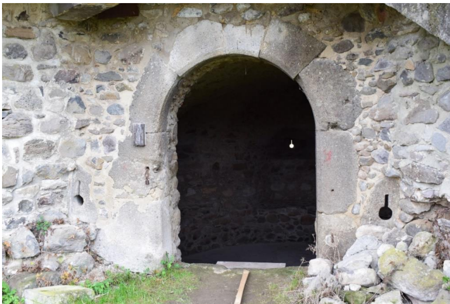
Figure 36 Negatively affecting adaptation elements: a) incorrectly reconstructed details b) invasive installation of engineering networks, c) reversible communication elements
