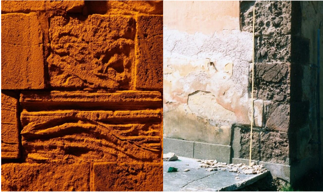
Figure 40 Effects of a) acid rain on the sandstone (Palma de Mallorca) and b) effects of salinization on the plaster and on the construction stone (castle tower in Banská Bystrica). Photo: Andráš, 2017, 1988
