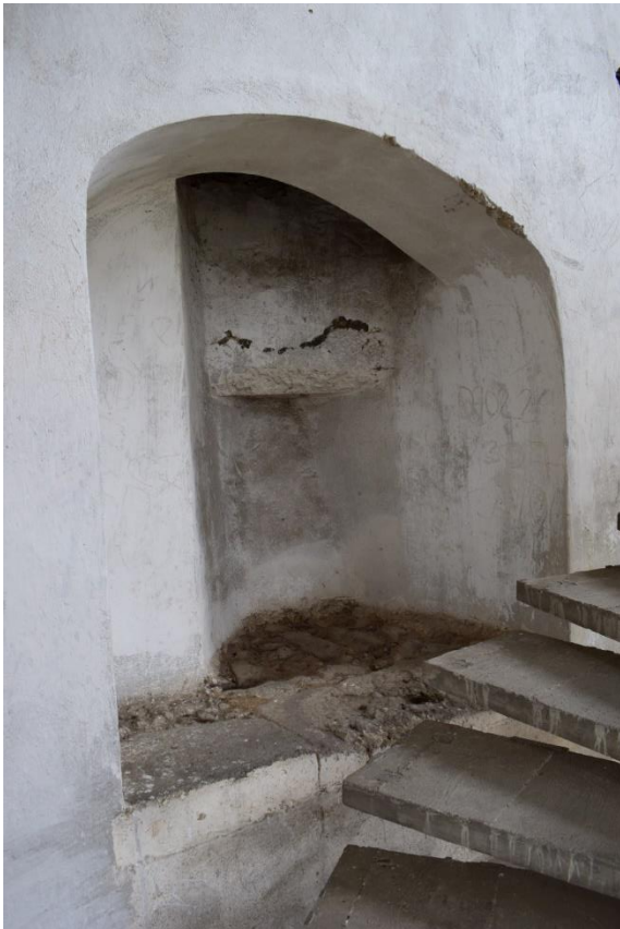
Figure 19 Northwestern bastion, the internal staircase in the masonry
