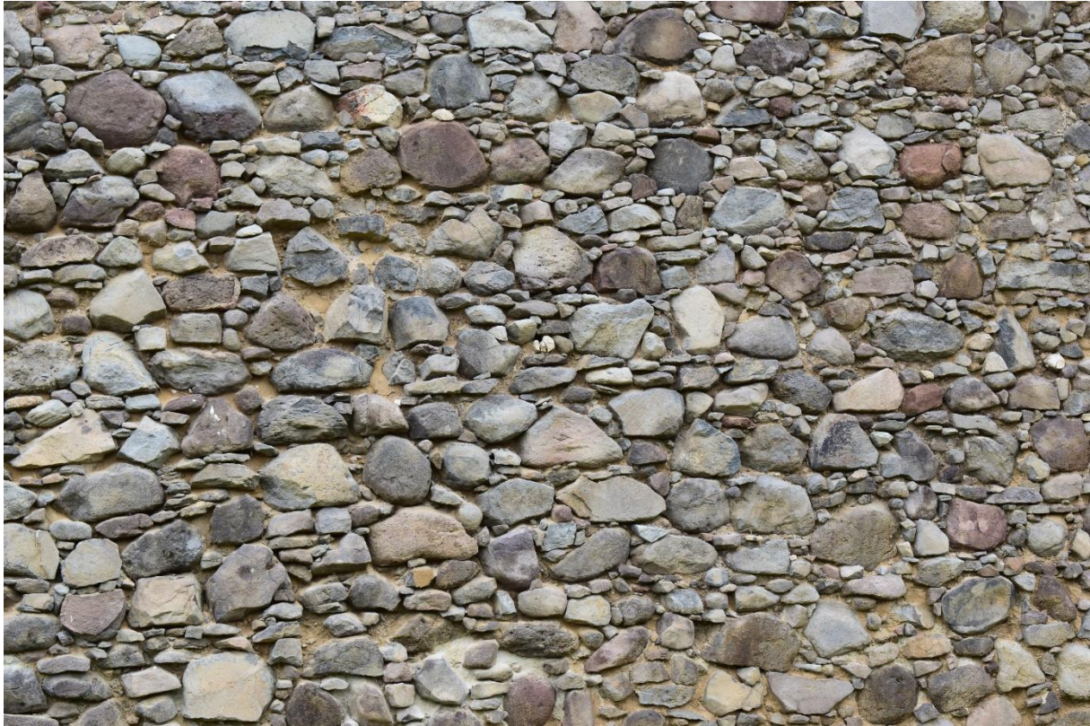
Figure 27 Quarry masonry from the quarry stone – the most common type of building structure
