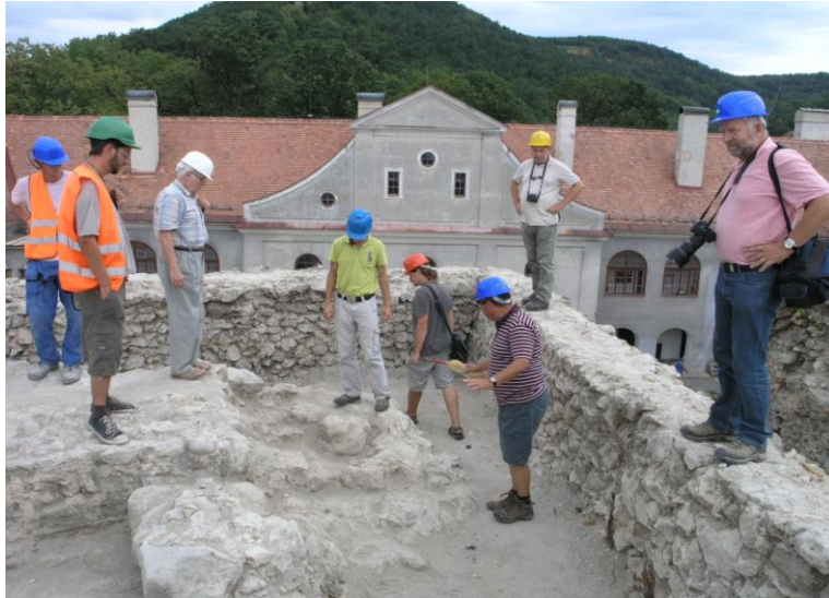
Figure 61 Precipitation water management at Castle Modrý Kameň. The proposal of underground drainage system leading the waters leaking through the ramparts of the ruin and causing its bad condition lead to a huge dig. Due to abundance of manpower, the digging pro
