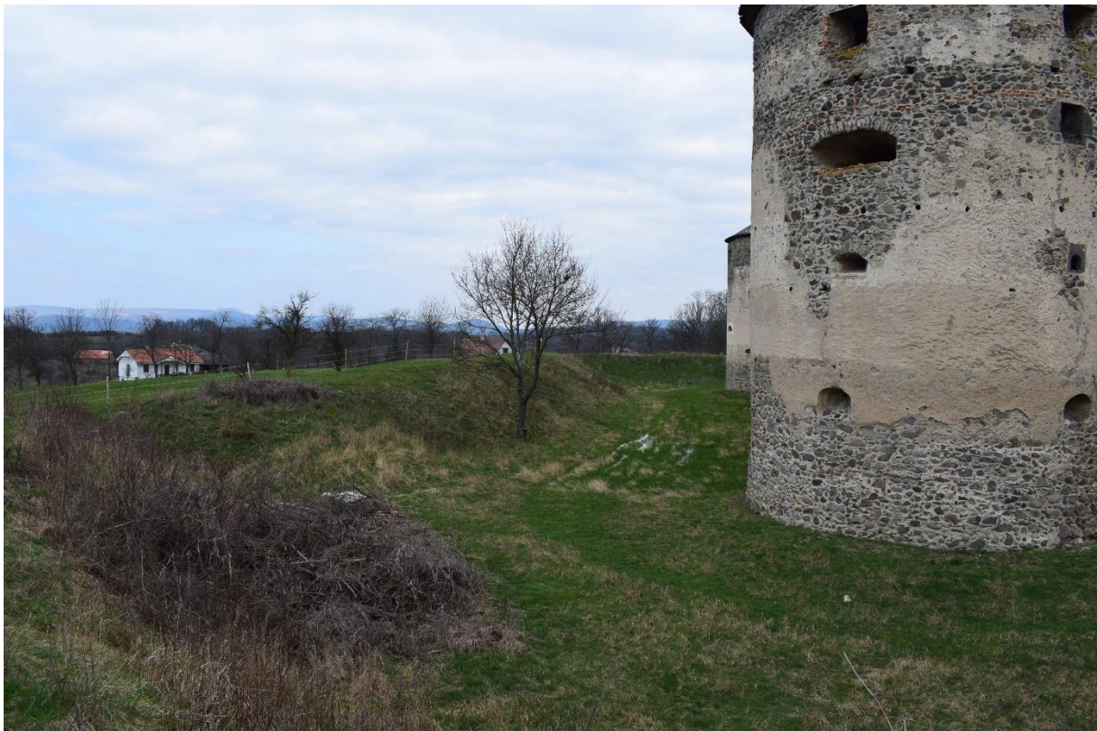
Figure 15 View of all lines of the fortification
